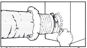
3. Pull jacket and insulation back over core. Tape jacket with at least 2 wraps of duct tape. A clamp may be used in place of or in combination with the duct tape.
